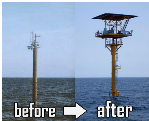
Before and after installation of deck, heliport and boat landing.
