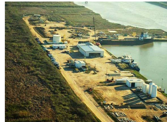
Aerial view of dock, fab shops and laydown areas.
